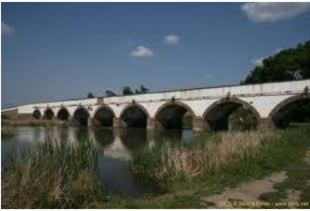
Nine Arch Bridge
